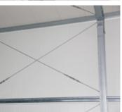
The interior is completely usable in height as the MEGAhall is assembled without traction ropes inside.
